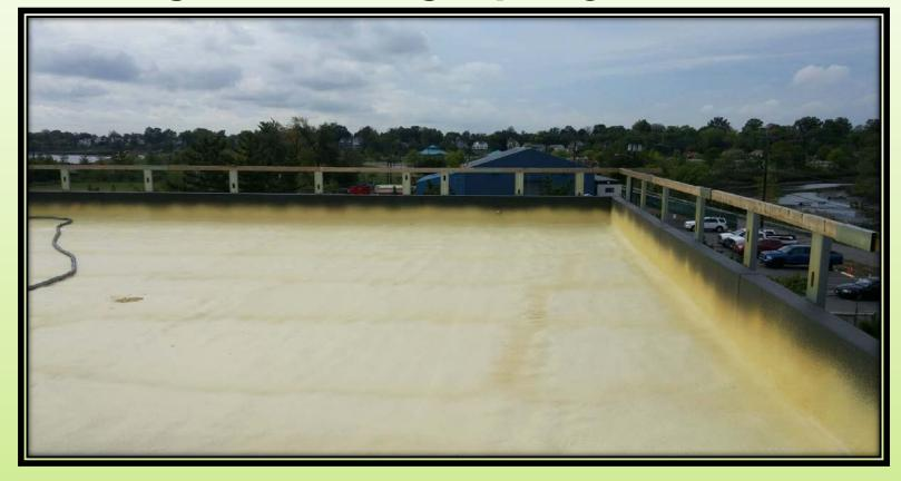
Spray foam effectively sealed and waterproofed the entire roof surfaces extending up and onto the parapet walls.
