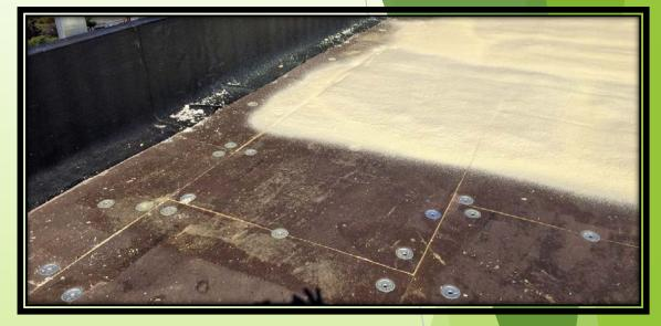
Plates and screws along with foam adhesive were used to install the tapered 5 cm / 2 in. insulation board.
