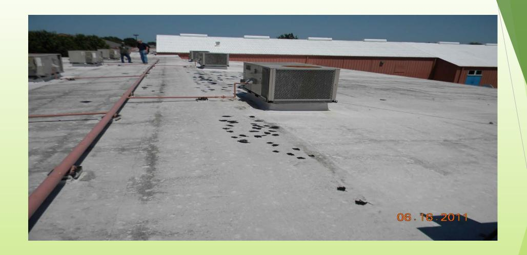
Overview of impact repairs on coated membrane with damage.
